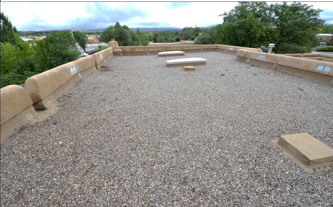
Flat Hot/ Tar & Mastic roof section with parapets on North Building.
