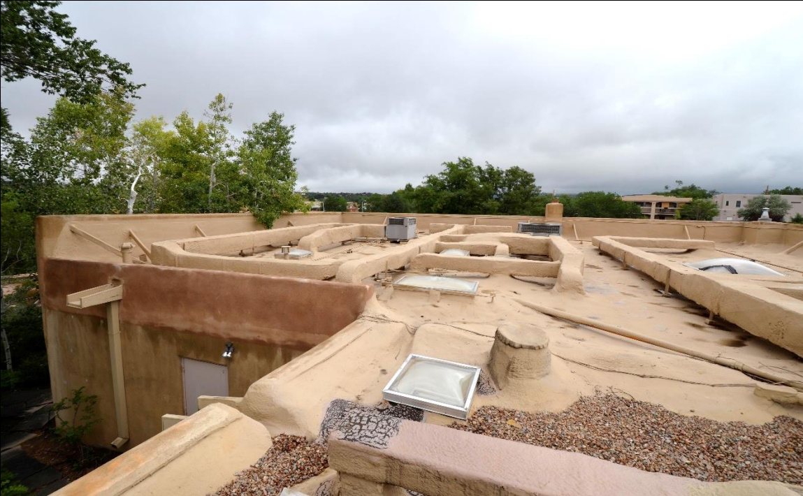
Flat Foam roof section with HVAC units & ducting on South Building.
