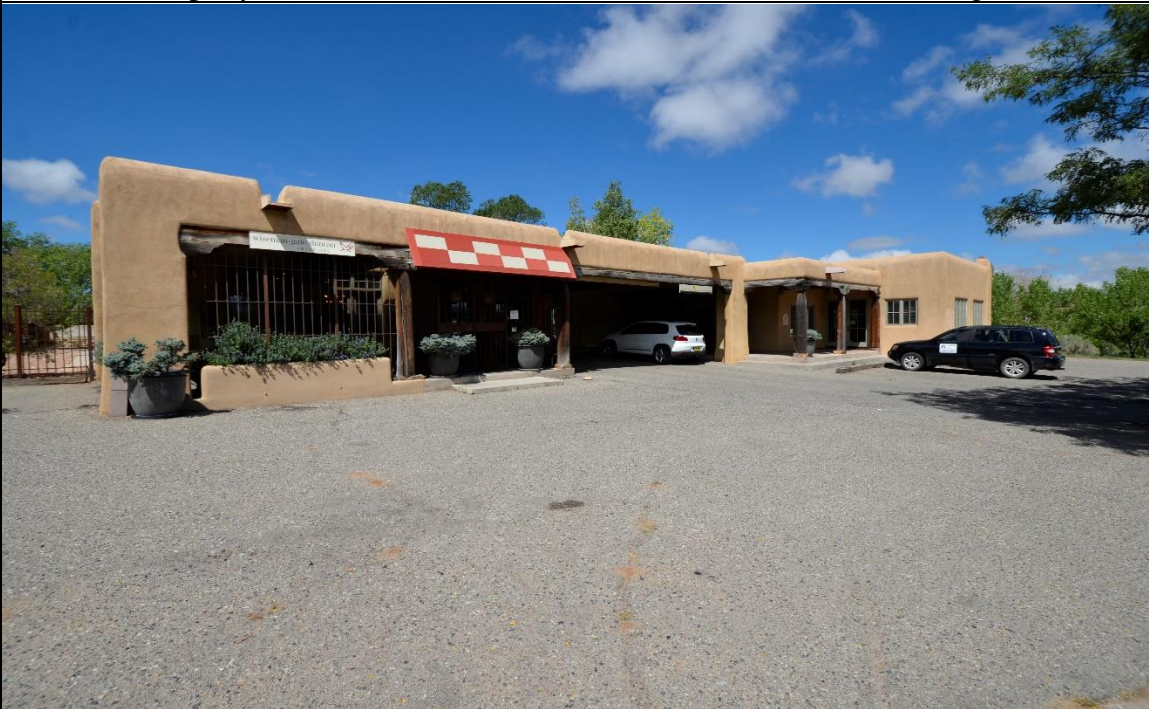
Property overview – East Elevation on the frontage of St. Francis Drive.
