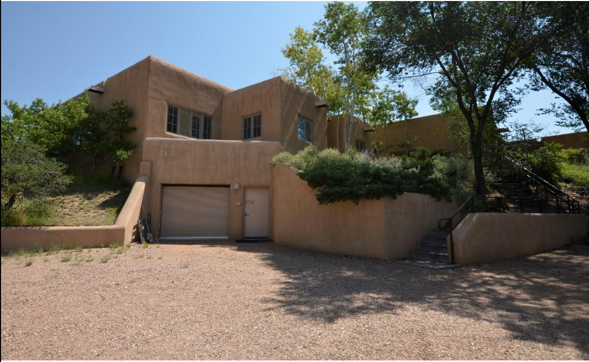
Property overview – North Elevation with natural surface drainage.
