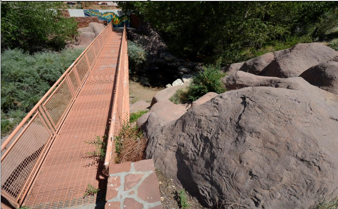
Stormwater drainage to the Santa Fe River basin.
