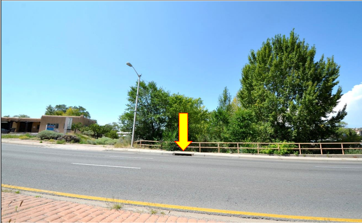
Stormwater drainage to St. Francis Drive culvert.
