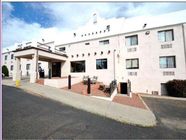
53. Entrance & Garden Level have exit doors that always remain unlocked and if locked should have an operating panic bar to be verified by the Fire Marshall.
