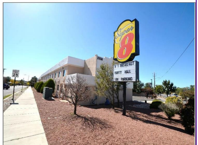
84. Street frontage and signage is in Satisfactory Condition.
