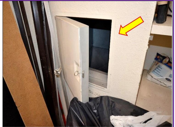
80. Two story Laundry shaft to Laundry room is not in use.
