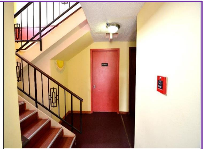
56. Staircase from the 1 st floor to the 2 nd floor are located at each end of the building with a middle staircase as required per fire safety codes.
