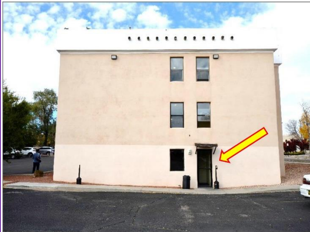
51. Garden Level floor South exit door should remain unlock and if locked should have an operating panic bar to be verified by the Fire Marshall
