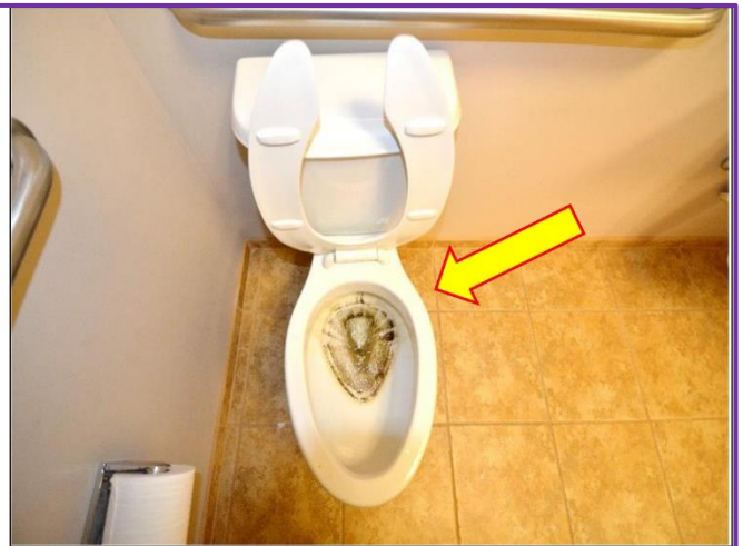
8. Sterling Toilet is badly stained and will need to be cleaned and/ or to replace if the stains are stubborn.
