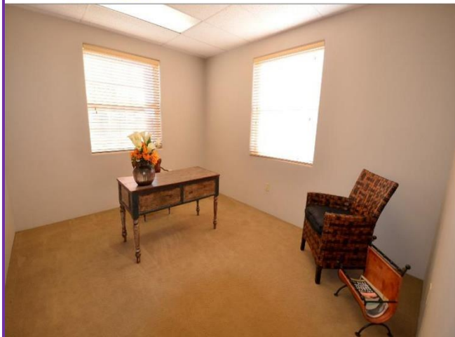
5. Office #3 with carpet floors, diamond plaster walls and acoustical 9' drop ceiling is in Satisfactory Condition .
