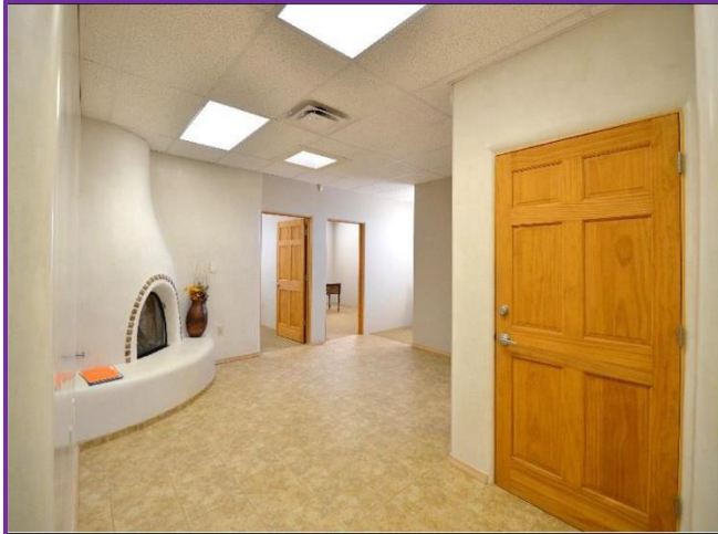
1. Reception Area with gas Kiva Fireplace, ceramic tile floors, diamond plaster walls and acoustical 9' drop ceiling is in Satisfactory Condition .
