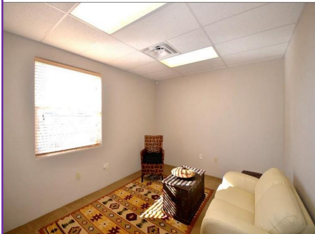
3. Office #1 with carpet floors, diamond plaster walls and acoustical 9' drop ceiling is in Satisfactory Condition .
