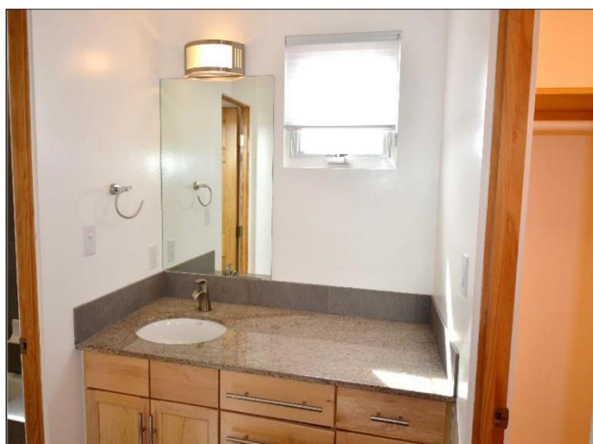
22. Upper Master Bathroom Vanity with 2cm Quartz countertop are in Satisfactory Condition .
