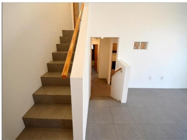
24. Upper and lower split-level staircases are in Satisfactory Condition .
