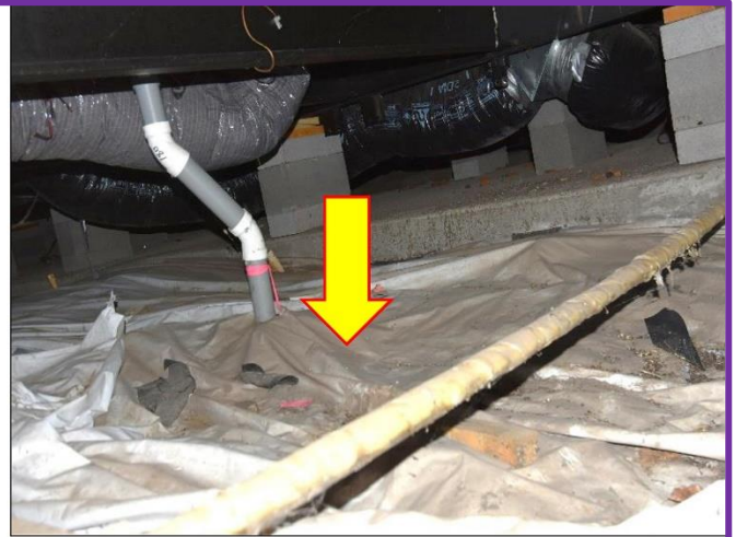
8. Crawl Spaces have plastic lining that will prevent Radon gasses.
