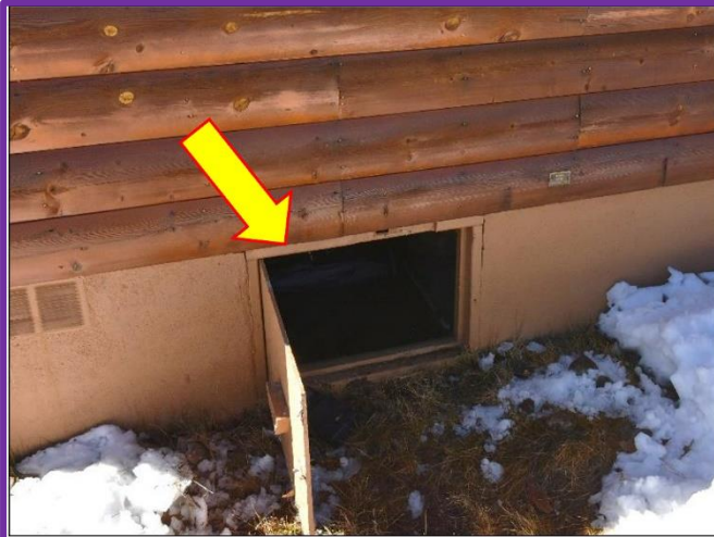
19. Single hatch found on both Modular Homes to access the Crawl Space.
