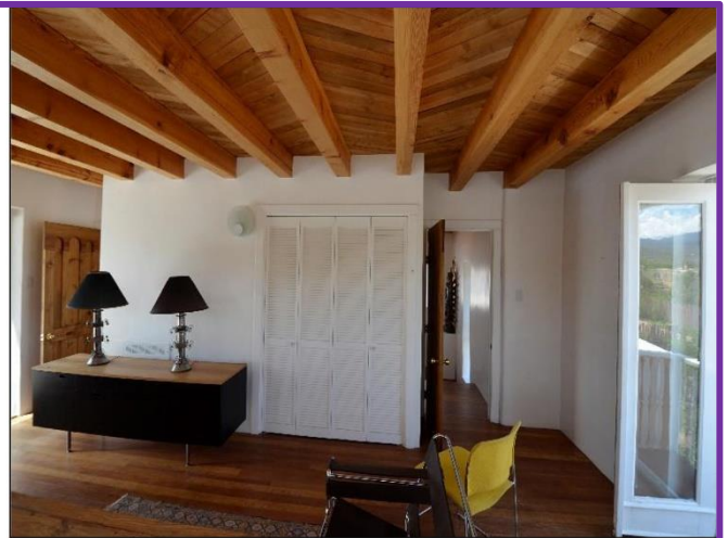
45. 2 nd Floor Bedroom with wood floors and beams with herringbone wood decking has a hydronic wall heater, not radiant in Satisfactory Condition.
