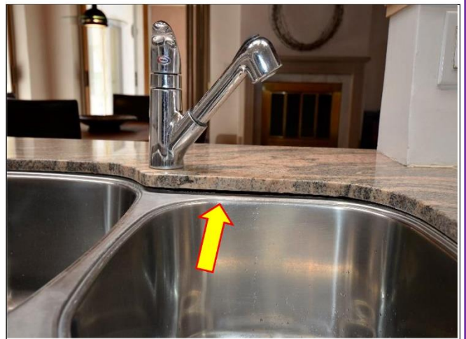
25. Granite countertop in Kitchen on the Main House and the stainless-steel sink are pulling apart, hence for the reason of an improper prop stick.
