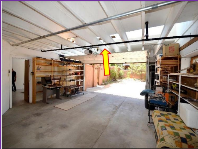
7. The piping below the Garage for drainage is too small in diameter to inadequate to drain the roof and could clog.
