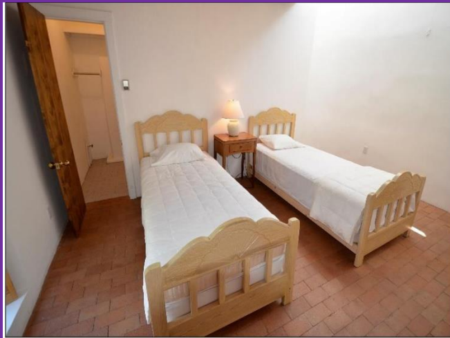
38. Bedroom at the end of Hallway is in Satisfactory Condition, with radiant floors that are working.
