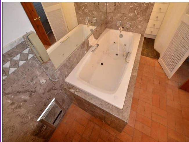
42. The Kohler Air Bathtub in the Master Suite Bathroom is working in Good Order and is in Satisfactory Condition.
